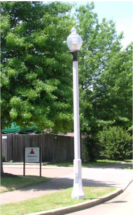
Standard concrete street pole with acorn head.
