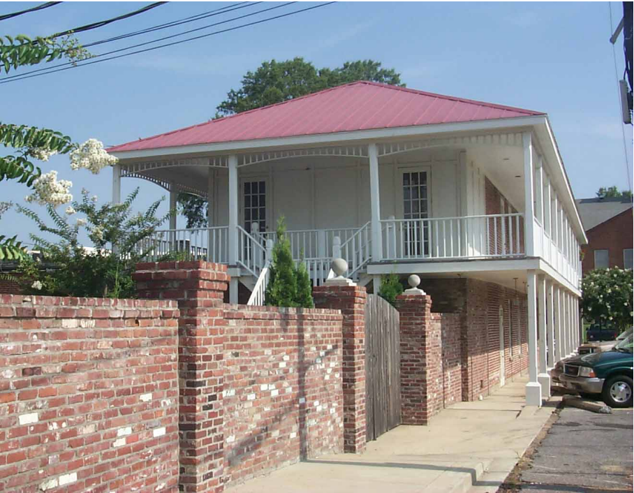
Porches can be the essence of the building.
