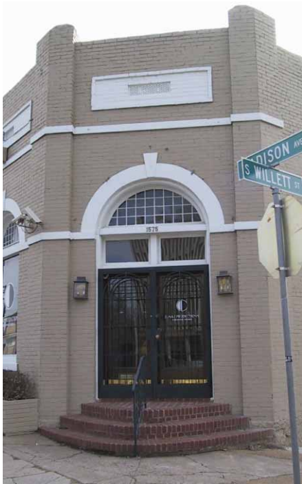
Corner entrance with stoop.
