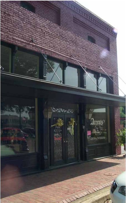
Large display and clerestory windows create transparency.
