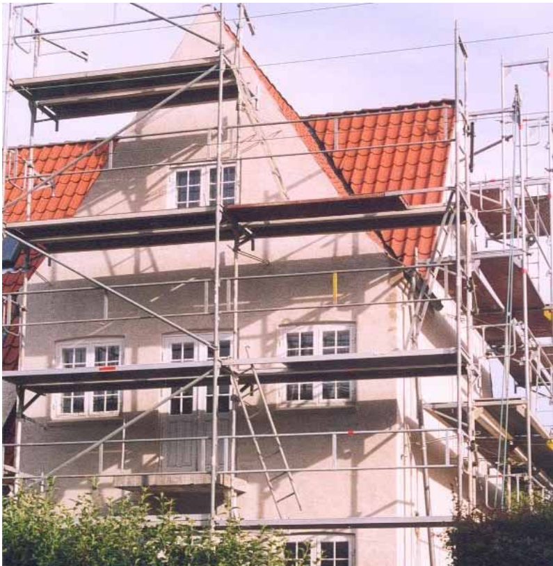
Most buildings can be made more usable through appropriate rehabilitation, rather than demolition and rebuilding.
