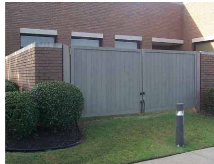
Bartlett City Hall screens its utilities.
