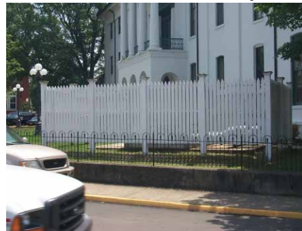
Screening should be in keeping with the architecture.
