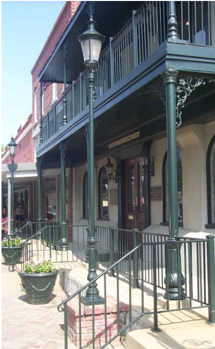
Cast iron porches.
