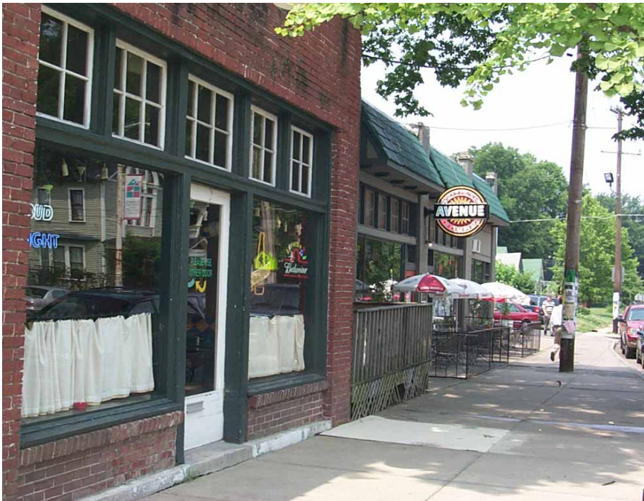
Maintain the front building line with fences or similar means.
