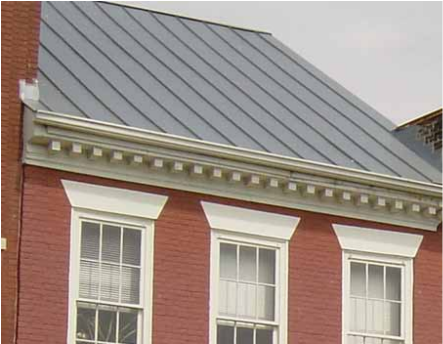
Brick Façade with Metal Roof
