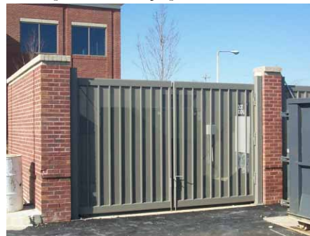
Opaque doors and walls screen dumpsters.
