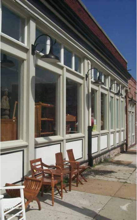
Lighting can accentuate the building.
