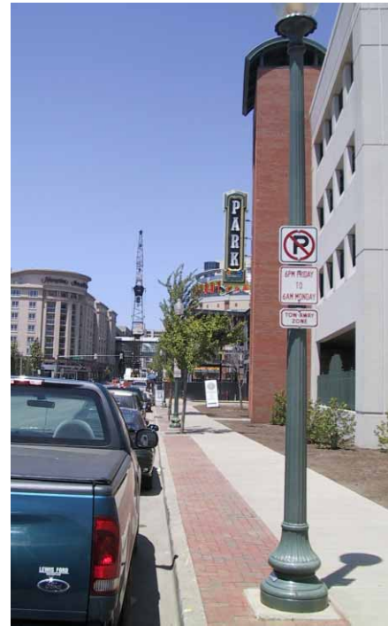
Brick used as an edge treatment.
