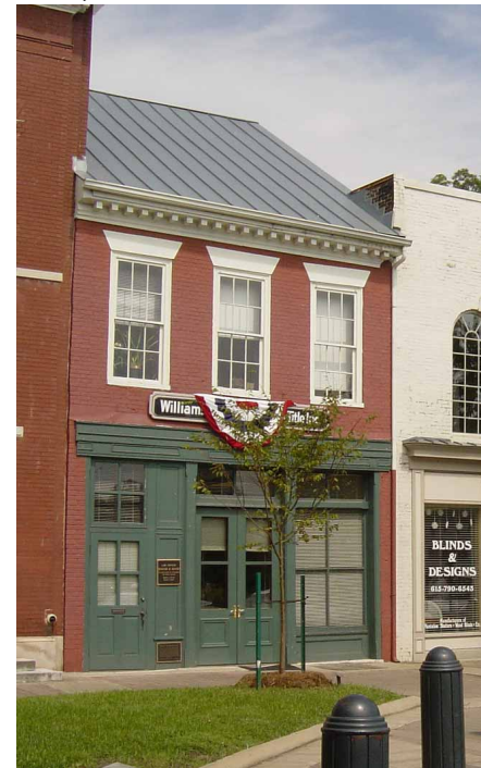
Sloped metal roof with decorated eave.
